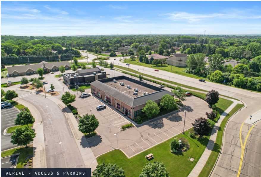
AERIAL • ACCESS & PARKING
